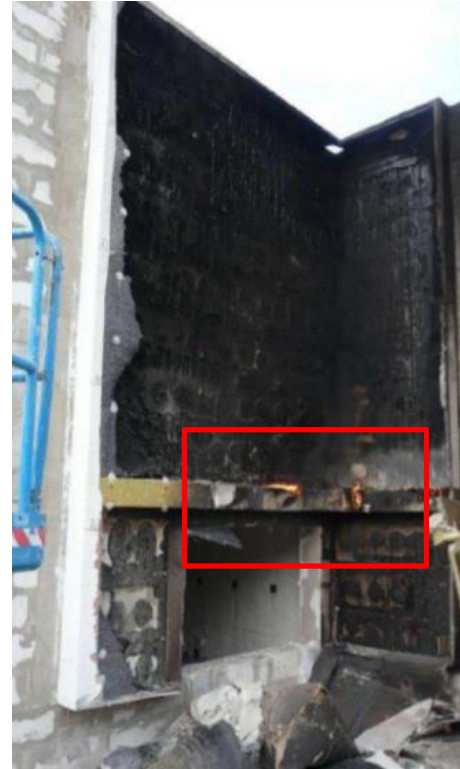
After termination of the test – the render system layer uncovered
