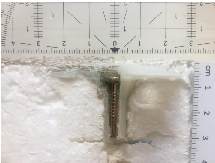
Real structure on the anchor (anchor plate cut open)
